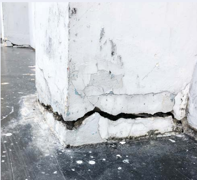
The second cracked pylon is structural, but poses no danger to the integrity of the main building, Mr Samrit said. Screenshot: Supplied
