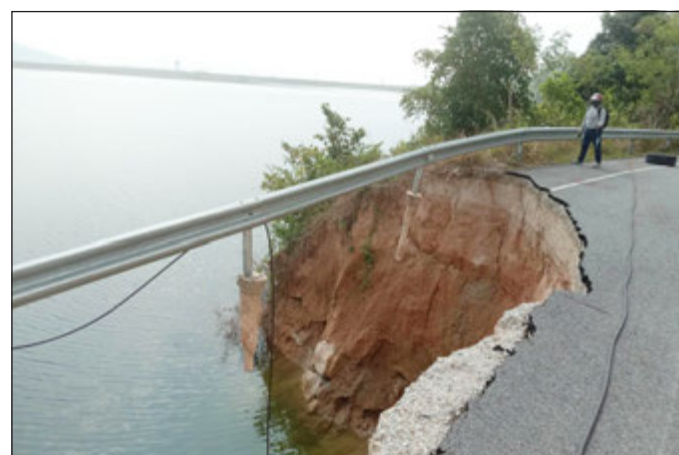
A large section of the road has collapsed into the lake. Photo: Eakkapop Thongtub
