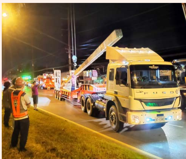
Work has begun on moving the power lines so construction of the underpass at the Heroines Monument can proceed. Photo: PEA Thalang / file
